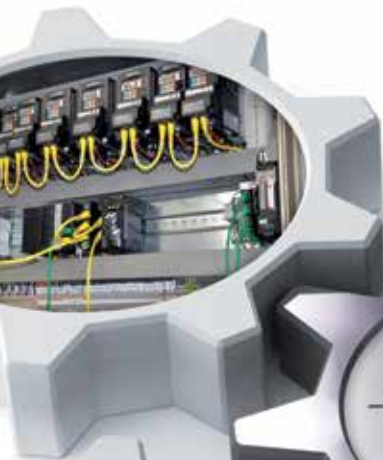
Panel builder / System integrator
